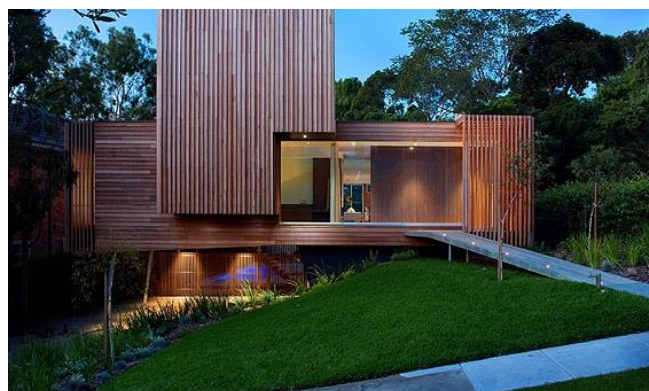
Radial Silvertop Ash screen boards and shiplap.
